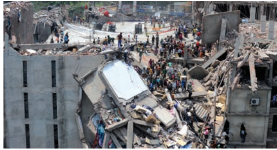
▲ The Rana Plaza building collapse in Dhaka, Bangladesh.
